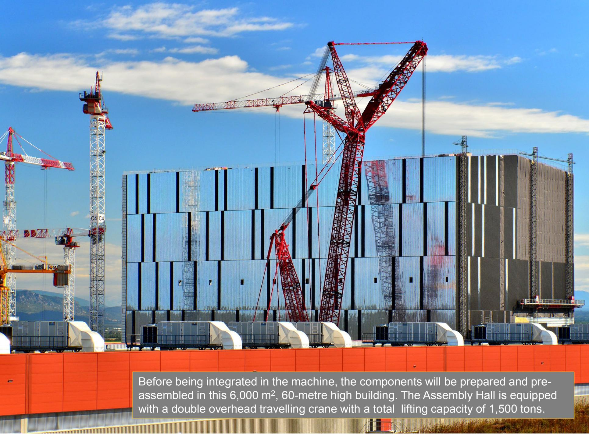
Before being integrated in the machine, the components will be prepared and pre-assembled in this 6,000 m<sup>2</sup>, 60-metre high building. The Assembly Hall is equipped with a double overhead travelling crane with a total lifting capacity of 1,500 tons.
